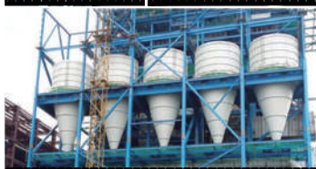
PULVERIZER INSTALLATION WORK AT KWDGI SITE
