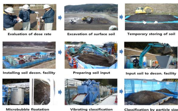
Fig. 2. Soil decontamination process in Japan.
