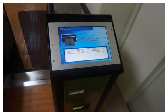
Fig. 2. PRIDE new access control system.
