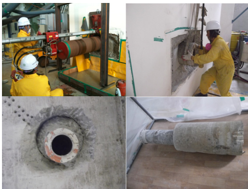
Fig. 3. Dismantling of beam port tube.
