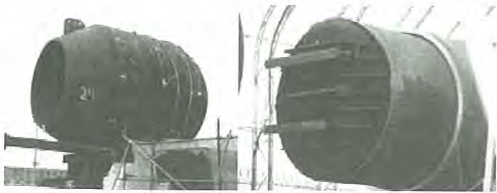
Fig. 2. Disassembled S/G (steam dome, lower part).
