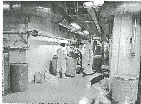
Fig. 1. Charcoal removal work with vacuum device.
