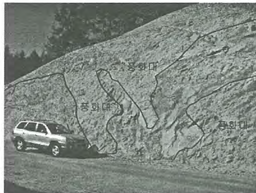
Fig. 3. Very irregular weathering contact at granite outcrop
